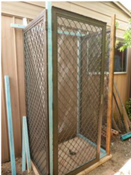
Framing using new structural pine and old security doors.
