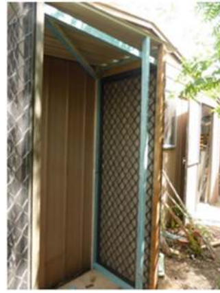
Scrap colour bond fencing used for sides and roof.
